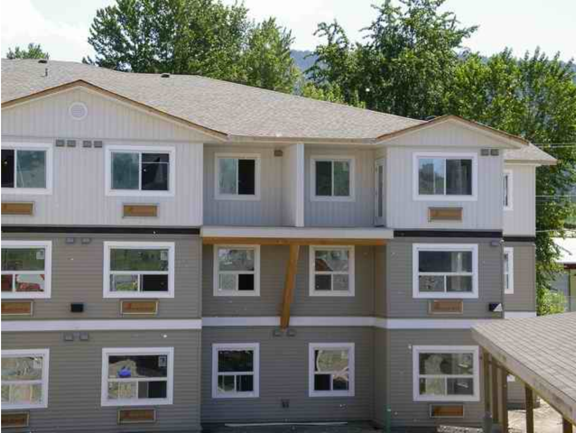
Heron Grove (under construction)
