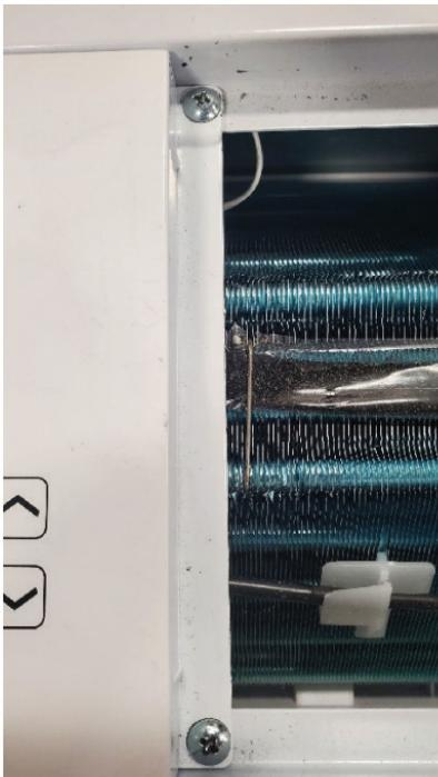
3. Gently remove the main control touch panel exposing the underlayment. Gently slide the underlayment away, take care not to disconnect any wiring harnesses, exposing two (2) mounting screws. Remove these and set aside to keep safe.
