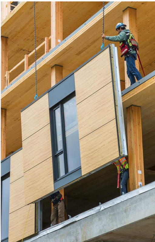
Example of prefabricated cladding panel installation [Brock Commons]
